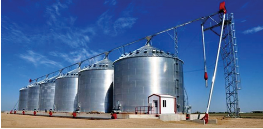
Installation of Grain Pump loop system into existing bin structure.
