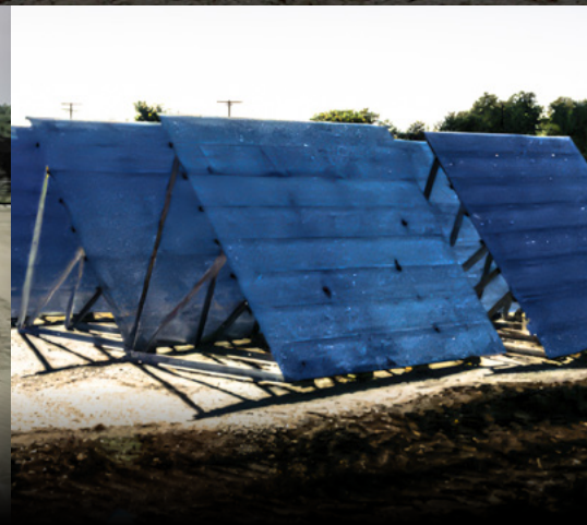
Modular design allows the system to be installed on slightly uneven surfaces in multiple configurations
