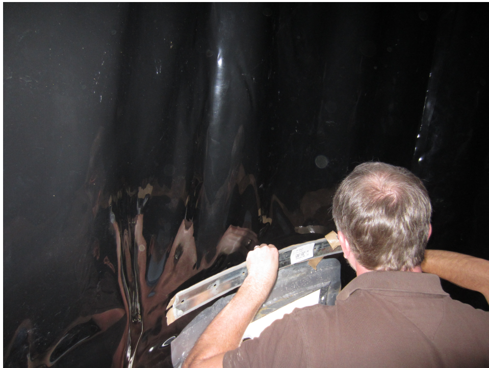
Figure 6. Access with liner clamps and trimmed liner
