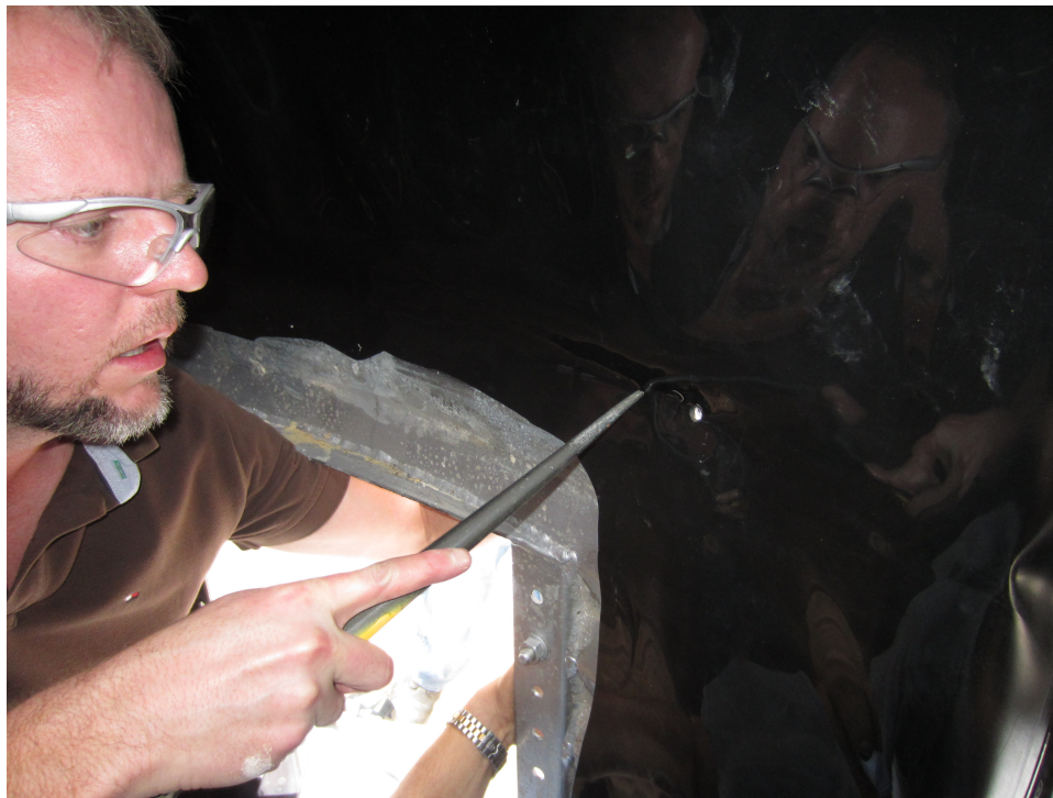
Figure 4. Punching holes through the liner
