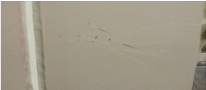
Figure 8. Scratches in Painted Surface
