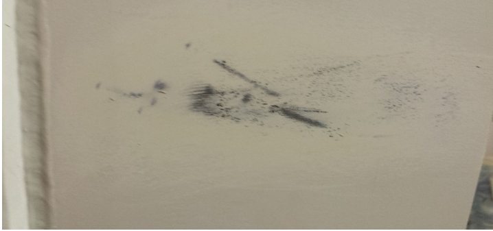
Figure 9. Nicks in Painted Surface
