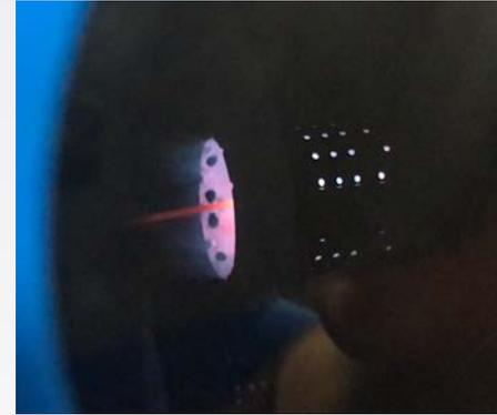
2. **Not enough air:** Take a look at the flame through the viewing window. If the flame has yellowish/orange tongues and is burning a bit further out the burner body, that is an indication that there is not enough air.
