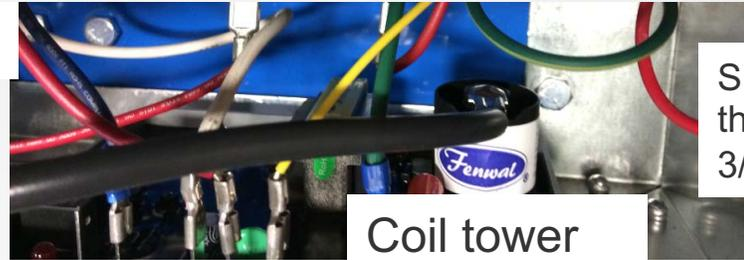
Slide the ignition wire off of the coil tower and hold it 3/16" from the coil terminal
