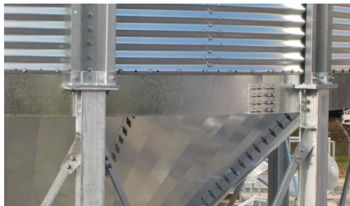
— Detail of the compression ring/leg/stiffener connection
