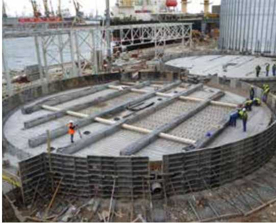
— Photo of aeration channel civil works
