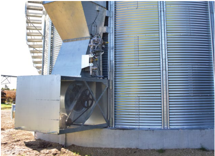
Ground-Mounted with Duct Work – The drying fan is mounted at ground level for ease of operation and maintenance. Duct work mounting directs the air to the drying chamber and creates an even heat and air mix.
