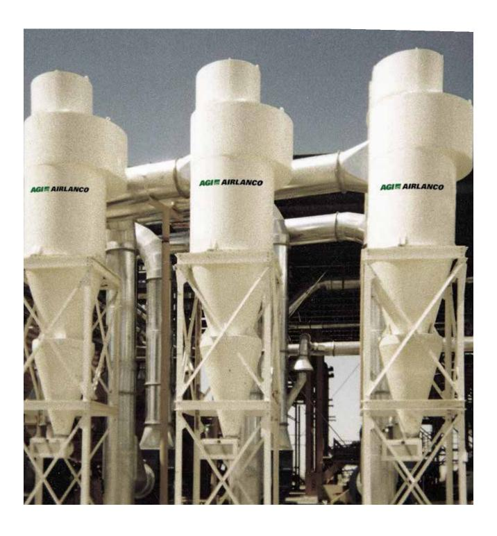
HE Series Cyclones provide high efficiency separation of dust and particulates from plant and process air. They can withstand high temperatures, moisture content and airflow. HE Cyclones are sometimes used as pre-filters to remove large, hot or moist particles that may damage filter media in other types of collectors. Their size is limited for maximum efficiency; consequently, HE Cyclones are often ganged to meet the demands of rather large air volumes.
