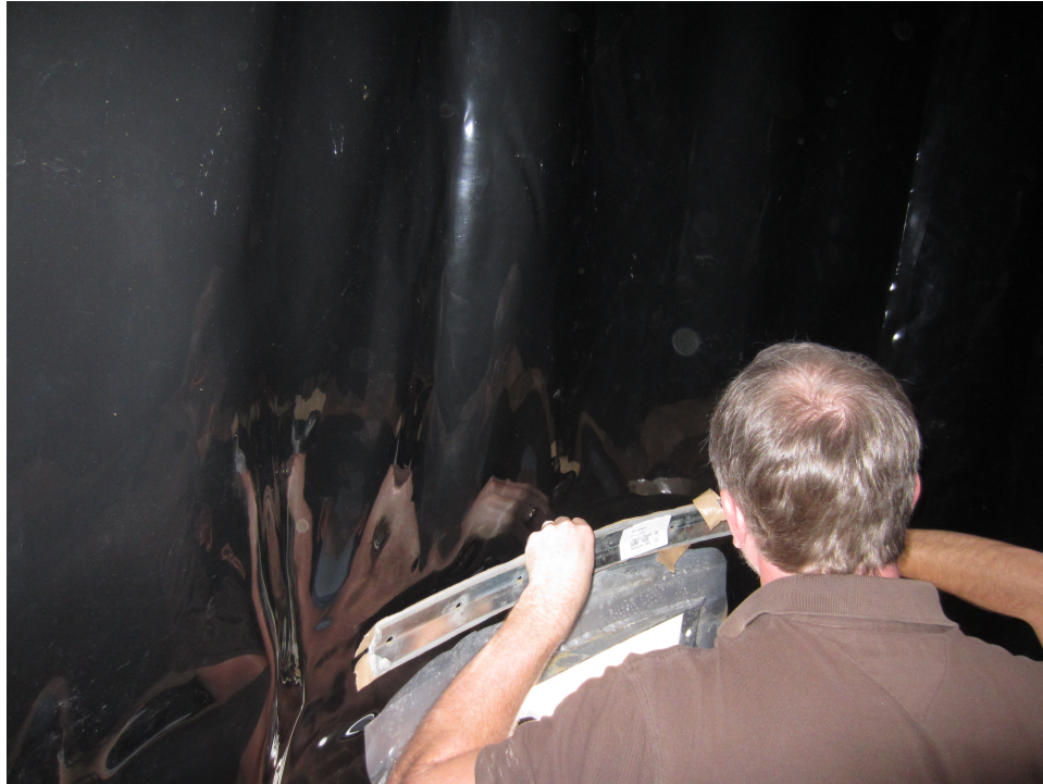
Figure 6. Access with liner clamps and trimmed liner
