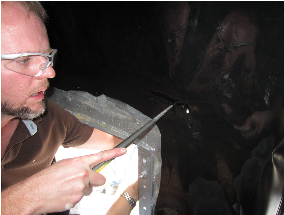
Figure 4. Punching holes through the liner
